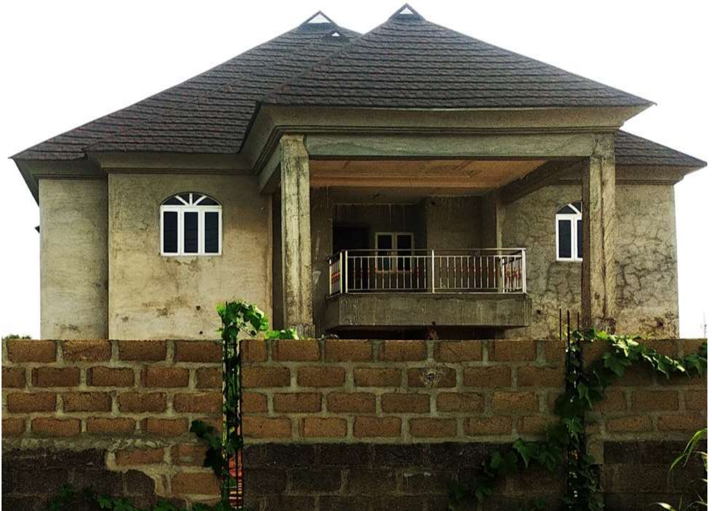
Figure 2: A Building and its Perimeter-fence constructed with Sandcrete masonry blocks as the major walling-material. However, while the Perimeter-fence is un-plastered, the Building is plastered with mortar as an exterior wall finishing-material.
