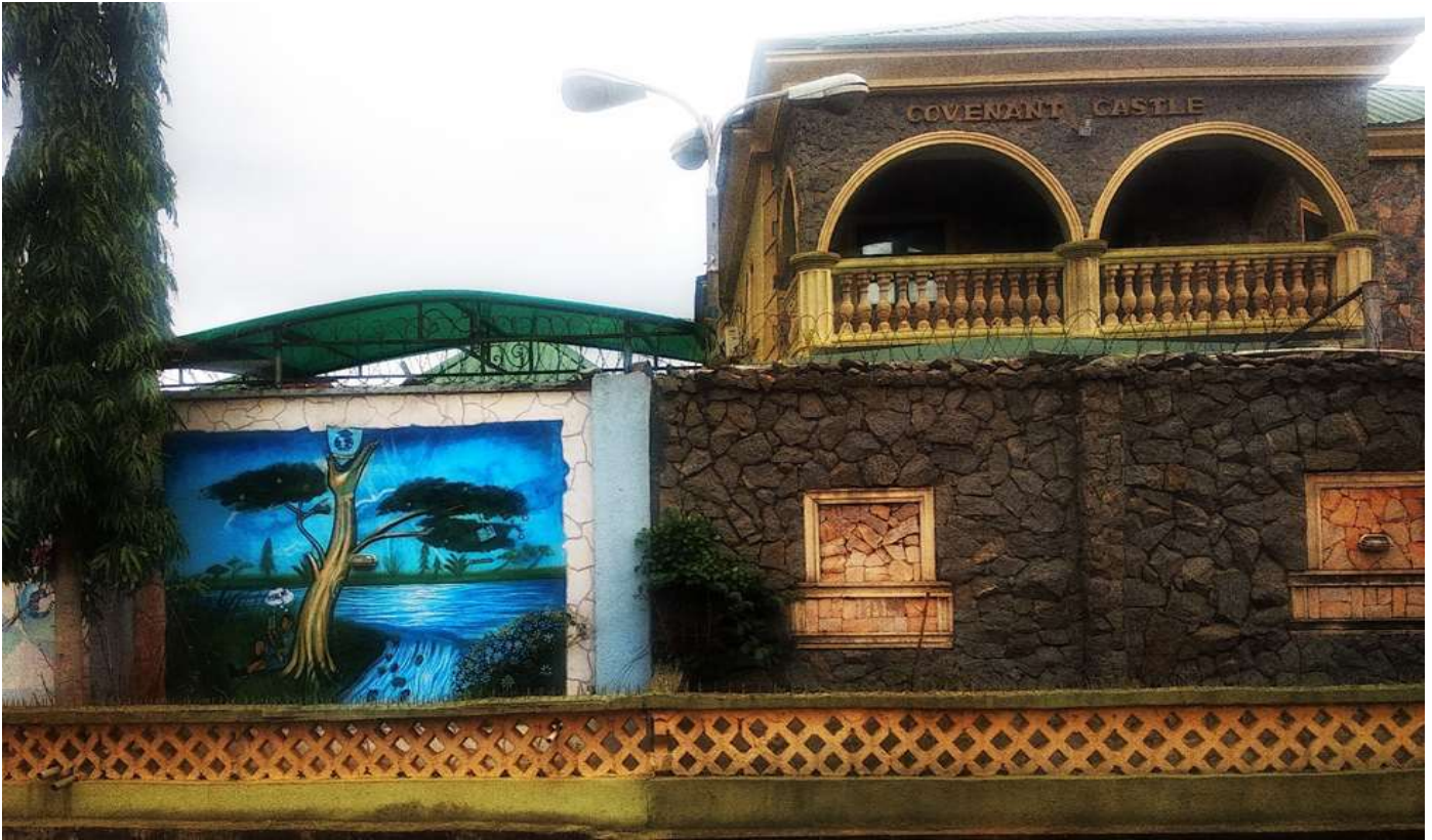
Figure 6: A Building and its Perimeter-fence constructed using Sandcrete masonry blocks and plastered with mortar. The exterior finishing of the Building and its Perimeter-fence is comprised of Painting, Painted art works, quarried Granite ('Hard core') stones and quarried Gravel stones
