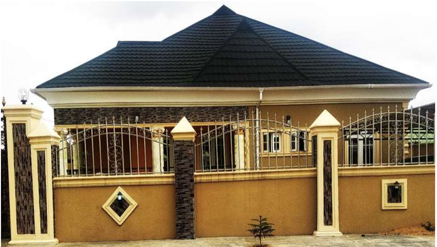
Figure 7: A Building and its Perimeter-fence constructed using Sandcrete masonry blocks and plastered with mortar. The exterior finishing of the Building and its Perimeter-fence is comprised of Painting and wall tiles
