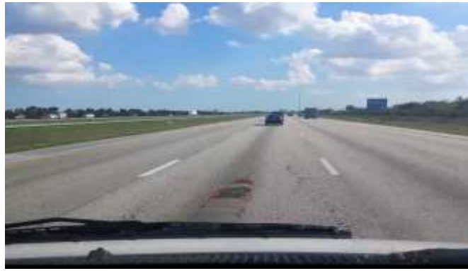
Figure 1: Sample frame saved by software to quantify the raveling
