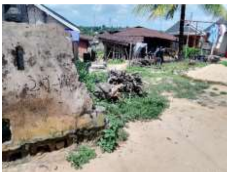
Plate 3: Substandard Houses/Environmental Decay
