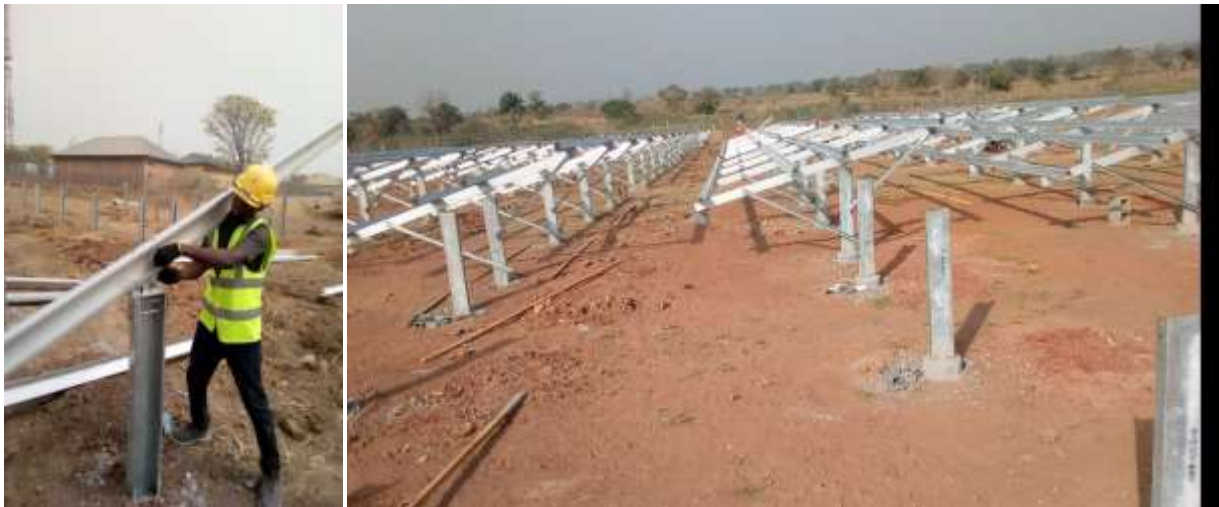
Fig 1: Installation of module mounting structure (MMS)
