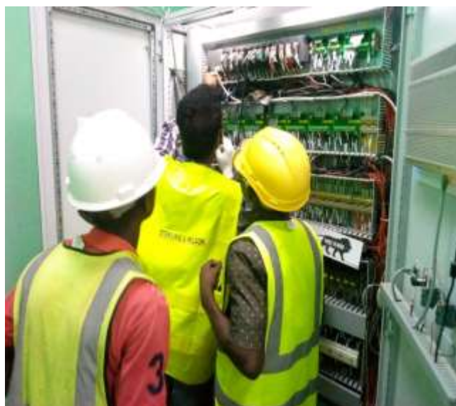
Figure 7: Installation of the SCADA system
