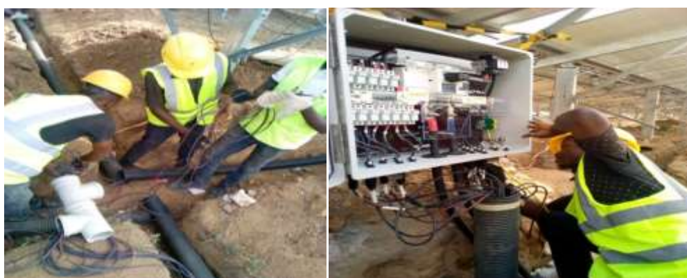
Fig 4: Installation and termination of cables at the SCB
