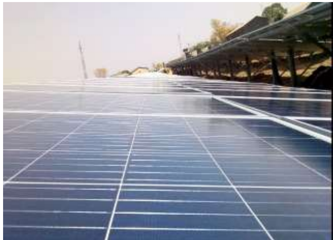
Figure 3: full view of an installed table
