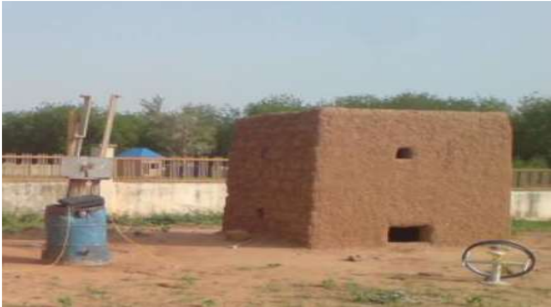
Figure 2.2 The constructed Adobe room
