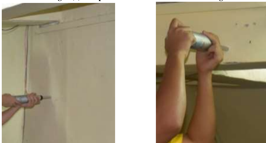
Figure 2. (b) Test by Rebound Hammer on Existing Members
