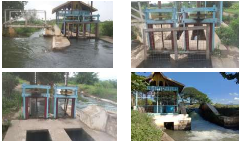
Figure 8. Lon Town Irrigation Channel at Madayar Township
