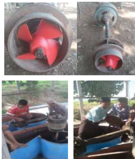
Figure 7. Installation Process of Turbine
