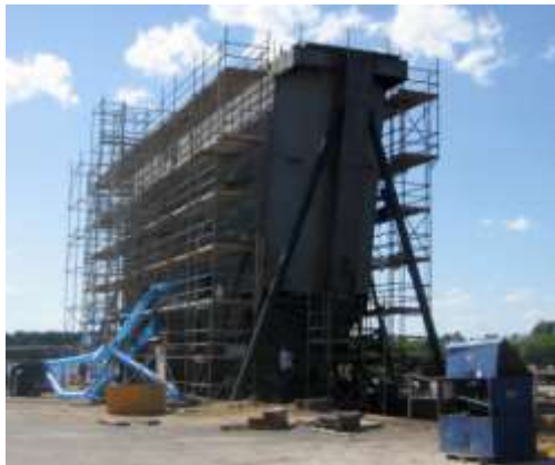
Figure 8: Dry dock gate under construction
