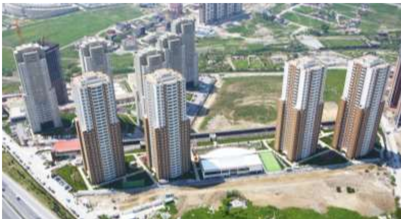
Figure 4. Air photo of Solar Kent
