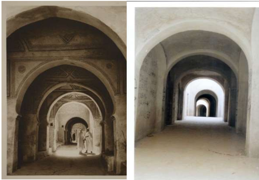
Figure 11: a picture of New Tamerna street in 1820 (on the right) and in the Ksar of Timasin in 1870 (on the left). The pictures show that the streets have sunny parts and shaded parts creating an artificial breeze in summer. [6]
