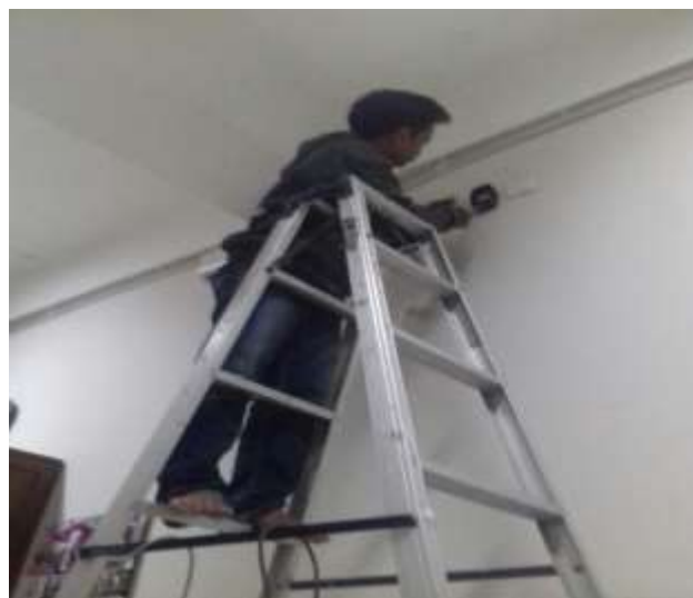
Figure 4.4: Installation of Motion Sensor for Air Conditioning System
