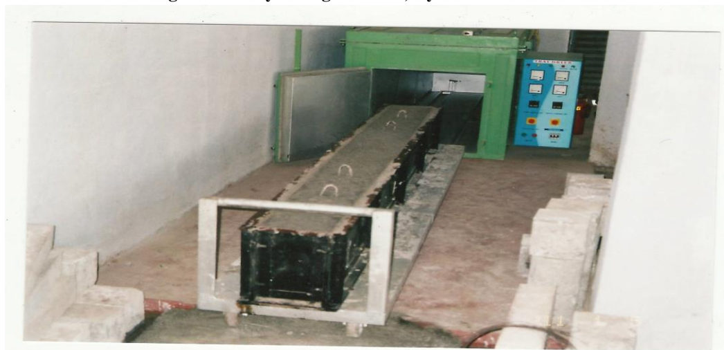
Fig.3. Oven dry curing of reinforced geopolymer concrete Beams
