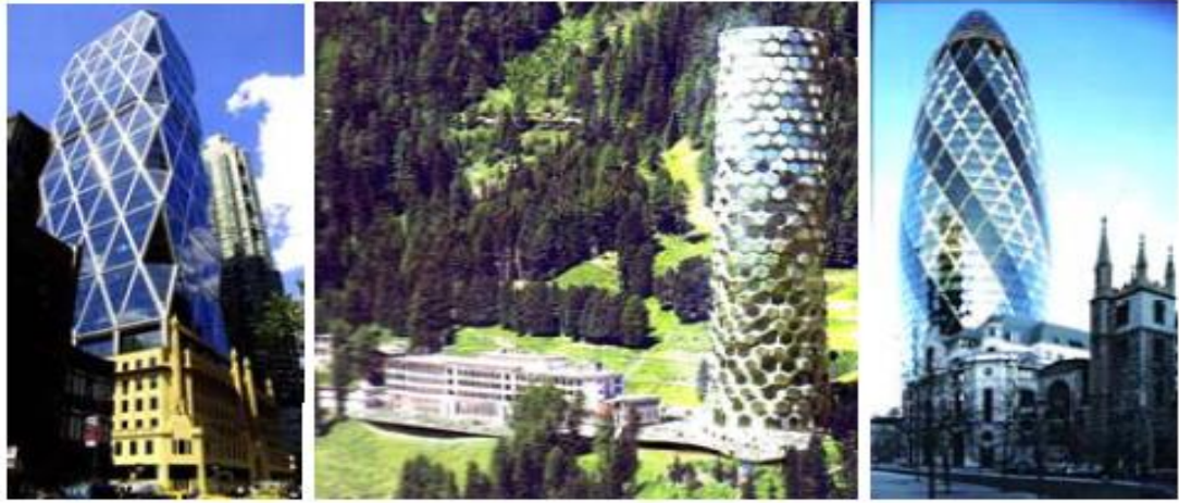
Figure 1: Hearst Headquarter in New York (left) Schatzalp Tower in Switzerland (centre) and St. Mary Axe Tower in London (right).
