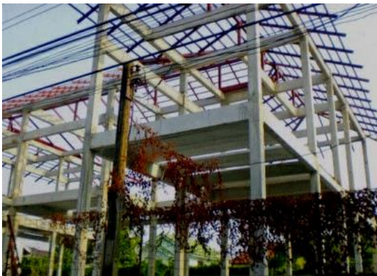
FIG 2: Precast Frame Systems [5]
